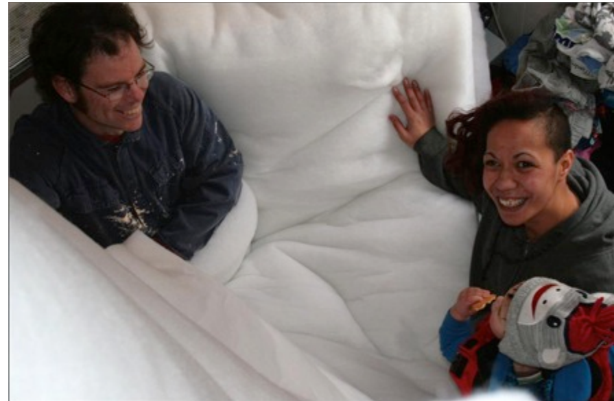
Transition Valley 473 member Alex King and resident Cassandra Thomas, with her nephew Hemi Birch (1) watch the new insulation go up into the ceiling of Ms Thomas' home. Photo by Dan Hutchinson from the STAR.
